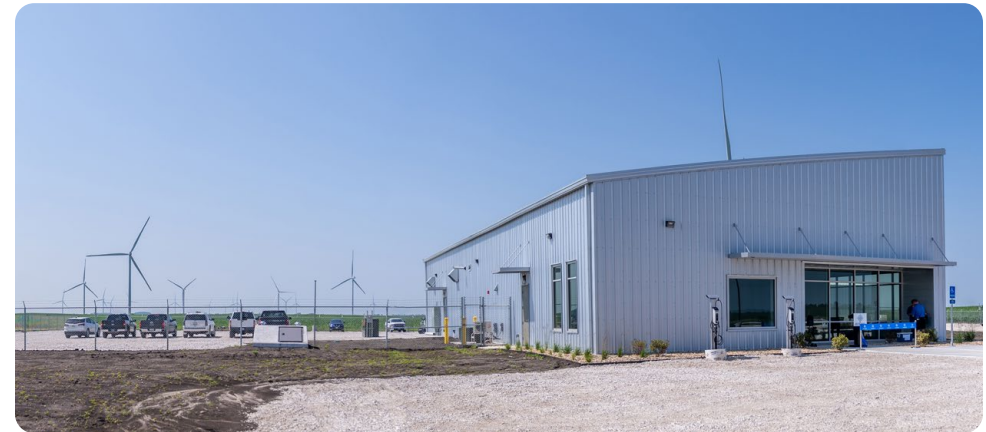
An energy-efficient operations and maintenance building at an operating Apex wind farm.
